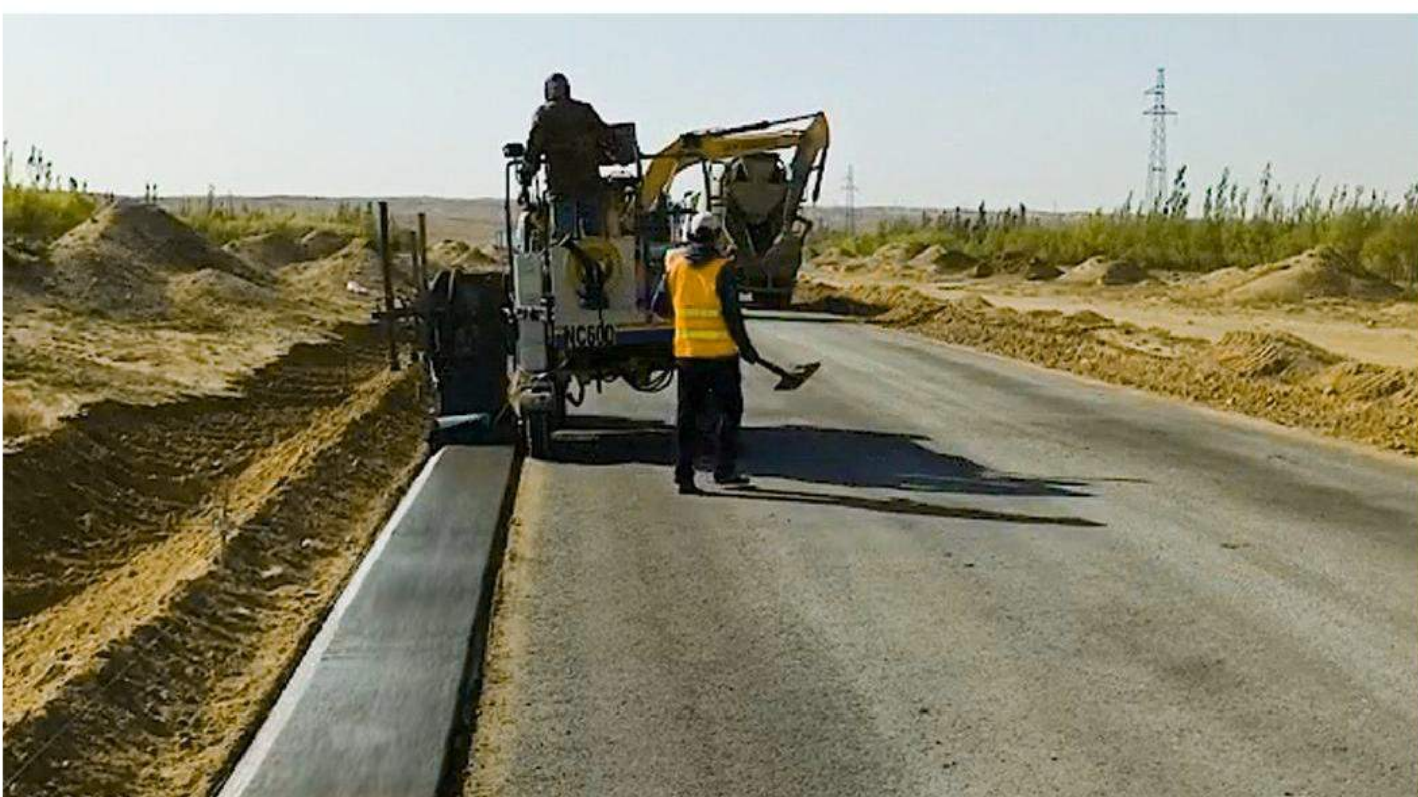
Slipform construction of Alashan shoulder in Inner Mongolia
