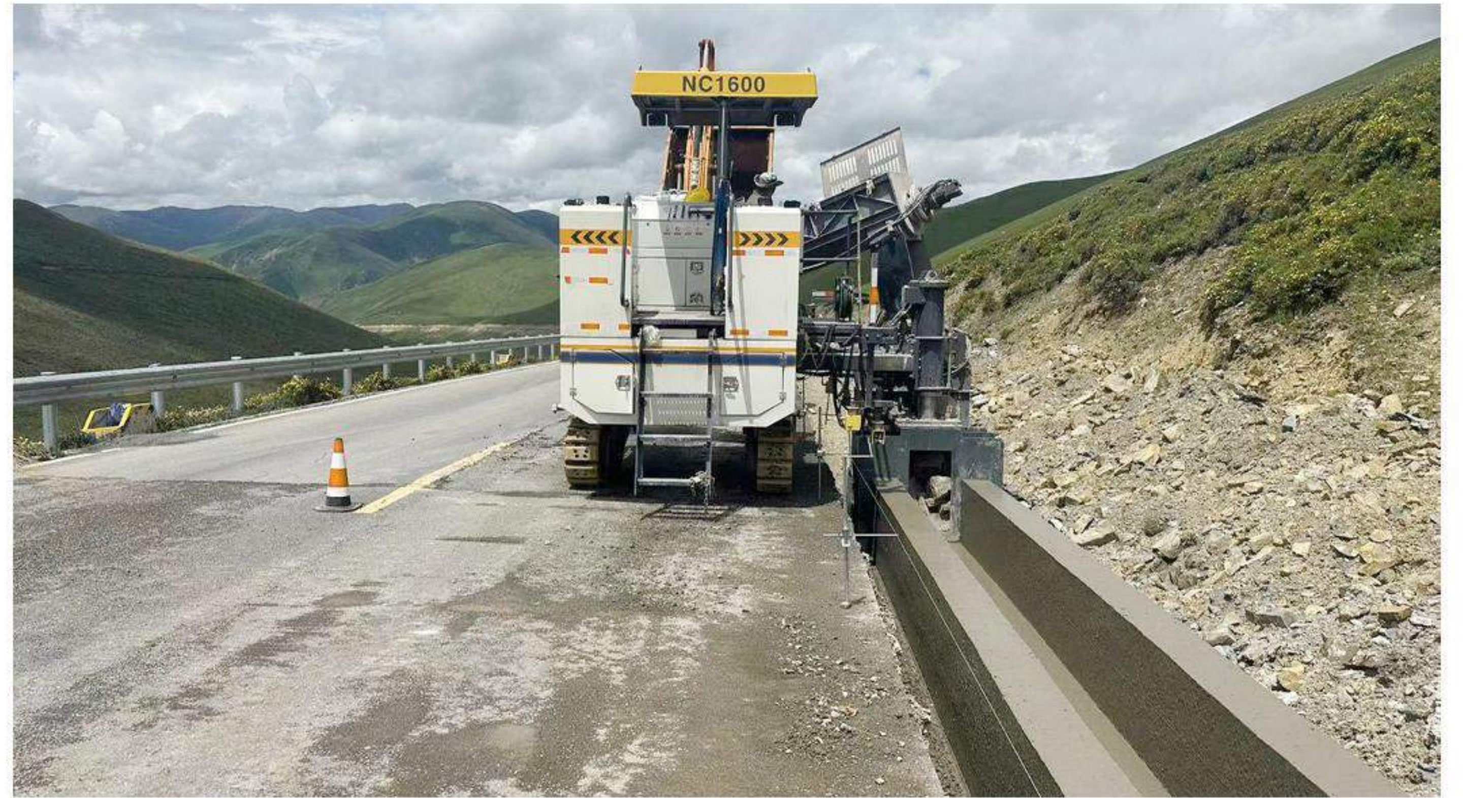
Sliding form construction of drainage ditch in Yushu City, Qinghai
