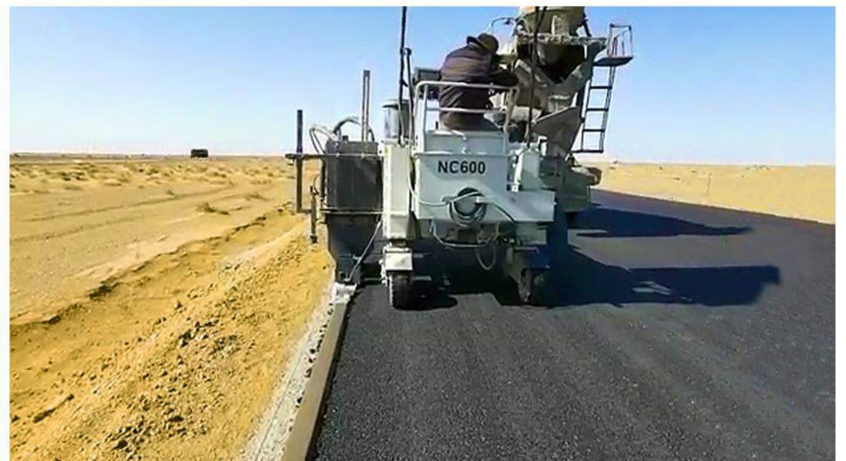
Slipform construction of kerb in Ejinaqi, Inner Mongolia
