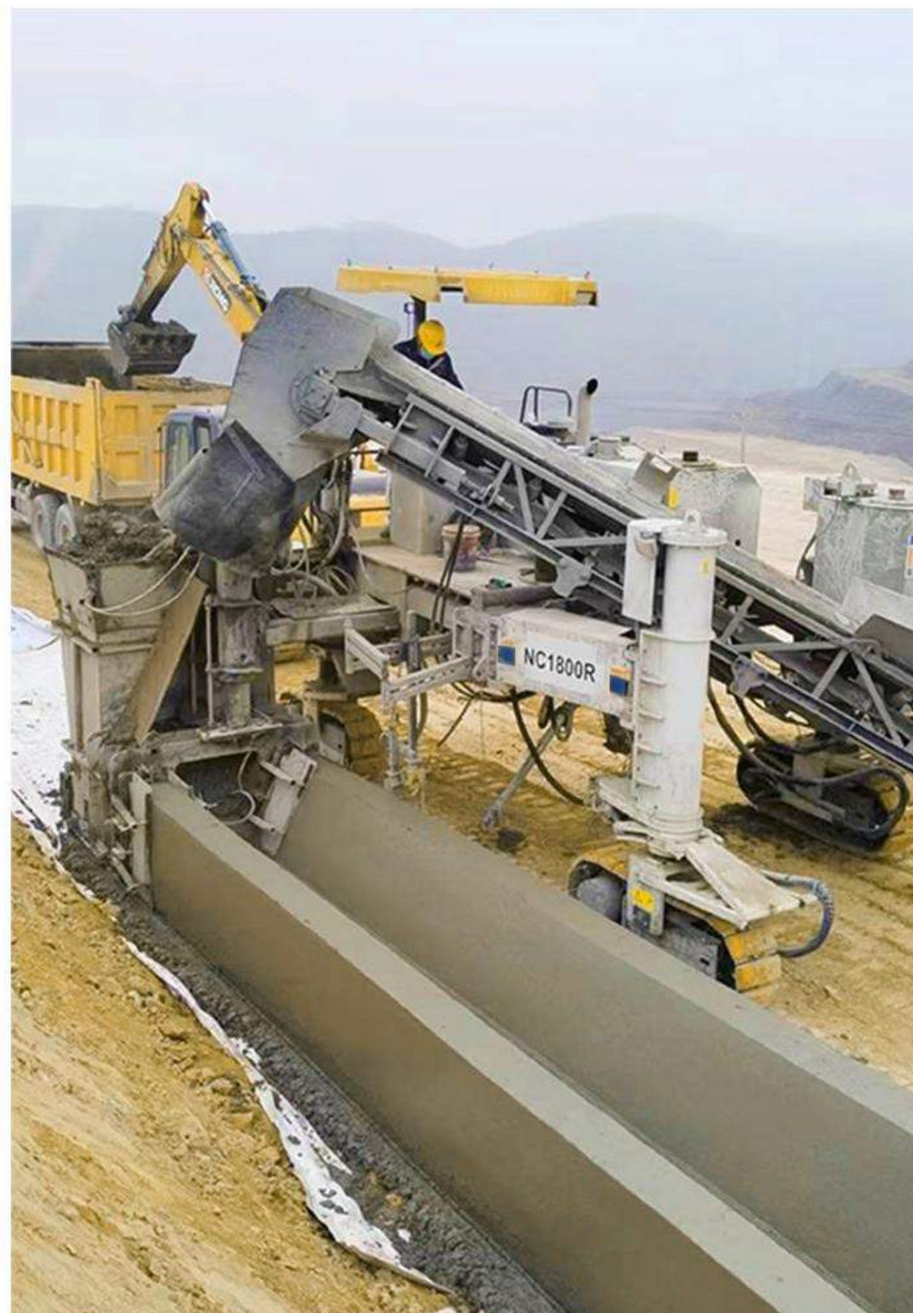
Slipform construction of drainage ditch in Guyuan, Ningxia
