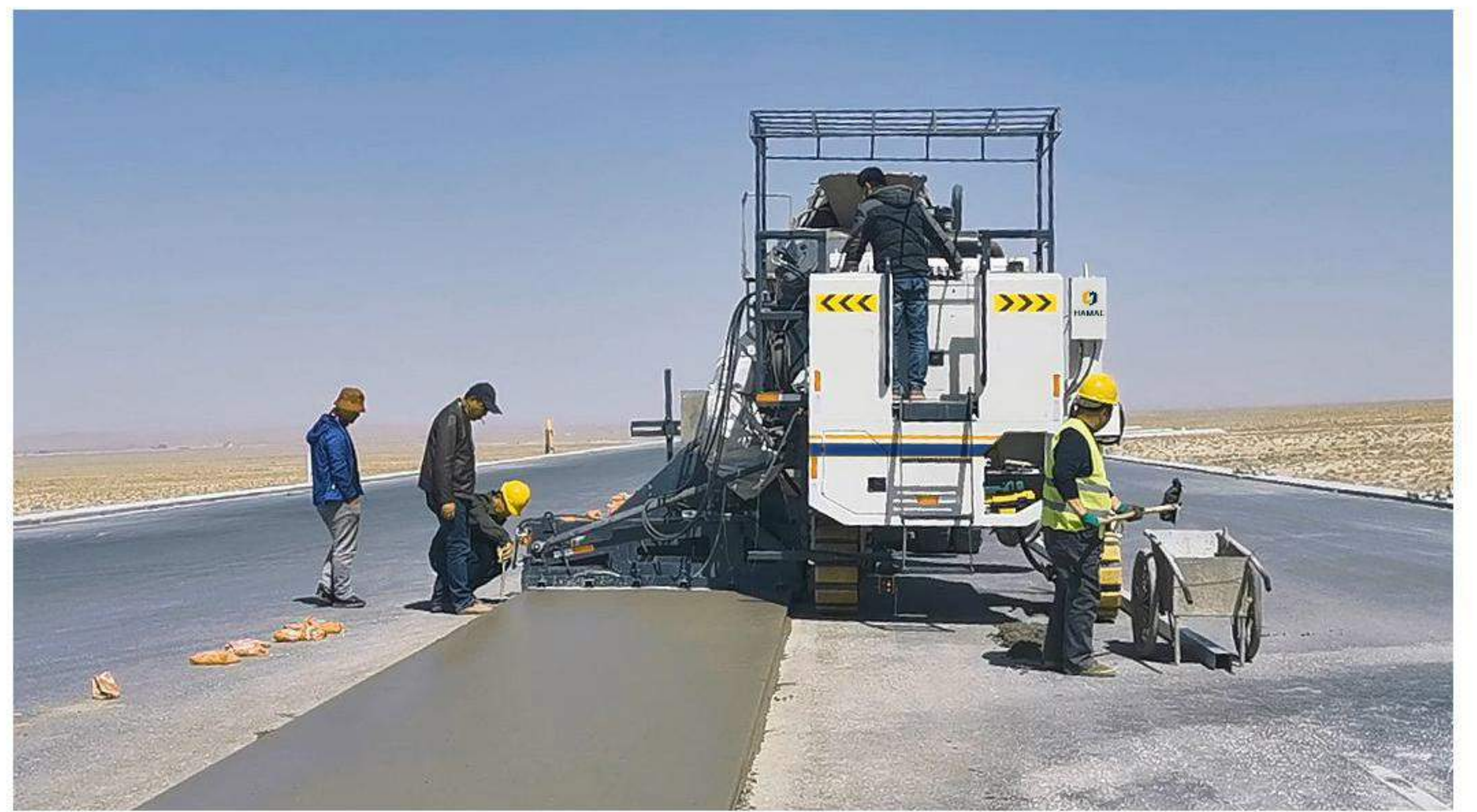
Slipform construction of Escape Room: Tournament of Champions meter wide shoulder of Dunhuang-Liuge Expressway in Gansu Province
