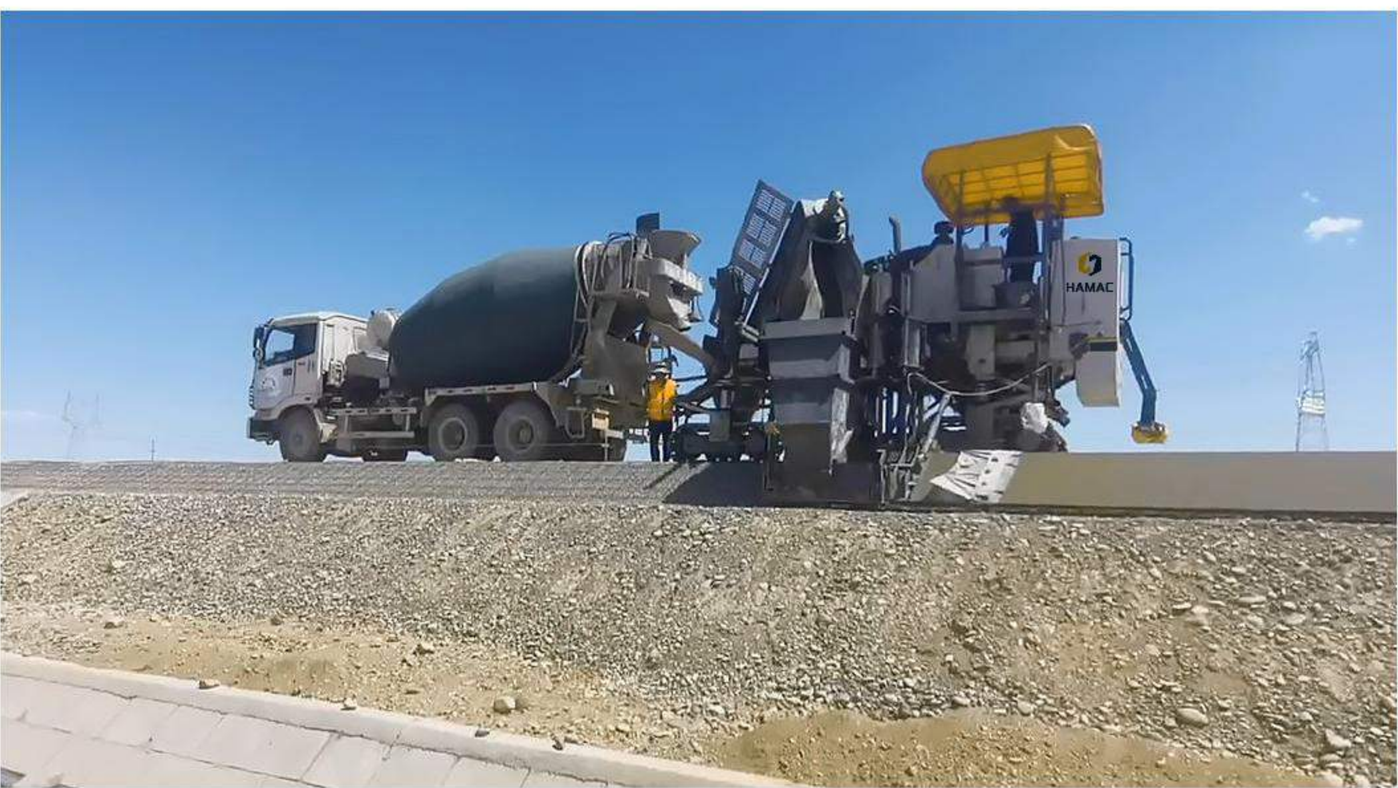
Slipform construction of hard shoulder in Jiayuguan, Gansu Province
