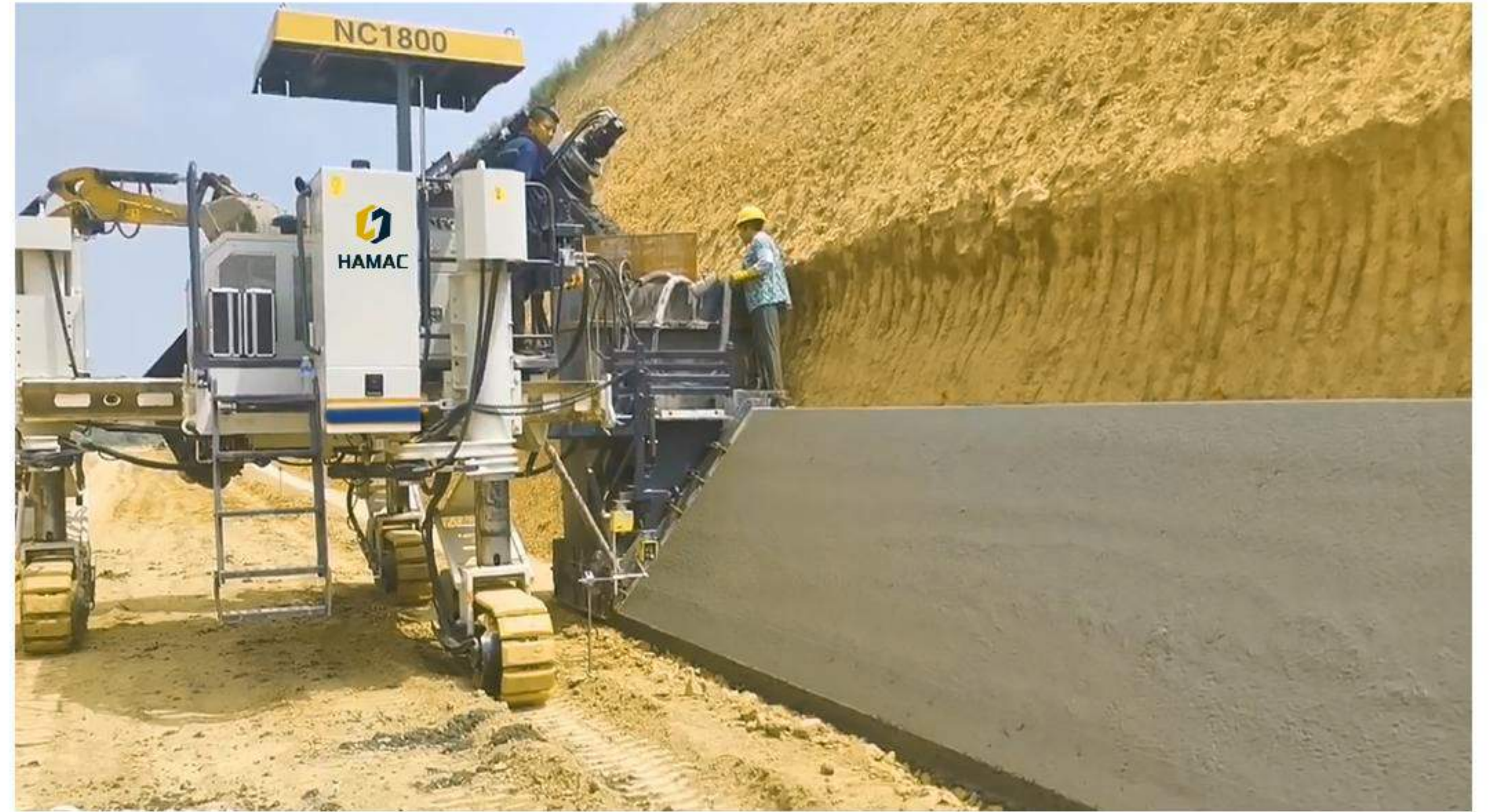
Slipform construction of retaining wall in Yuanping, Xinzhou, Shanxi
