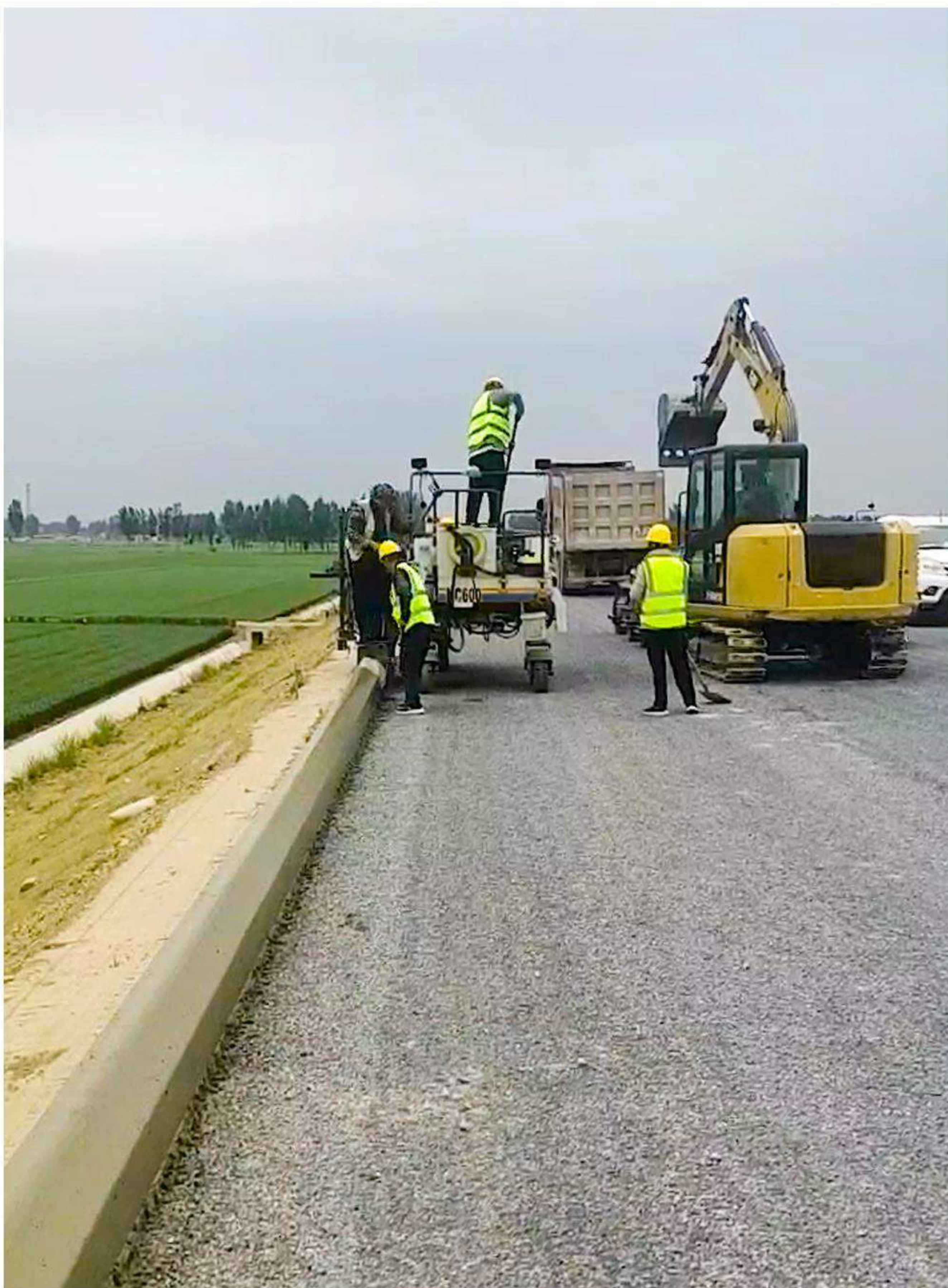
Slipform construction of curb of Yuanyang Expressway in Henan Province
