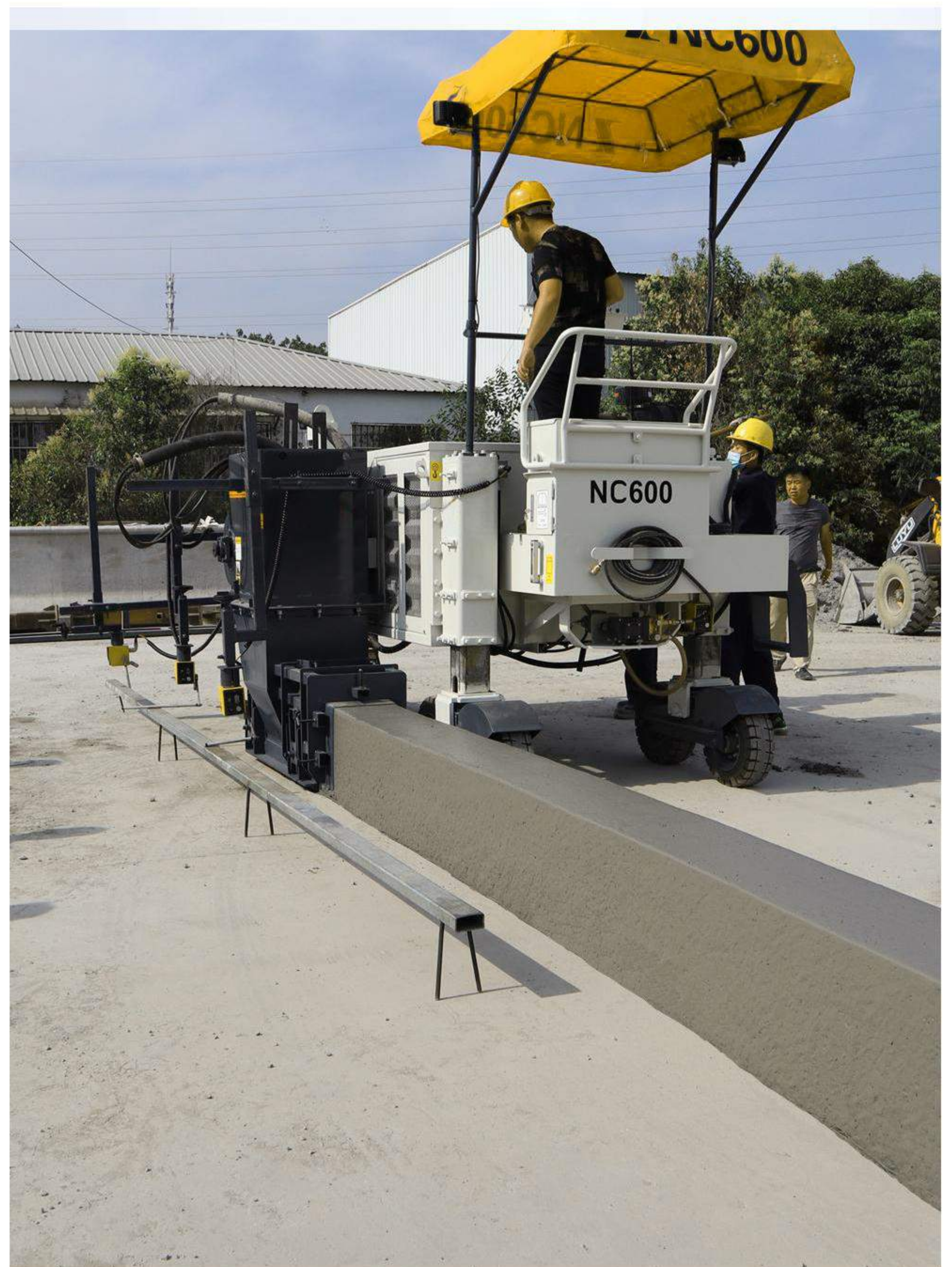
Slipform construction of small low wall in Maoming, Guangdong Province
