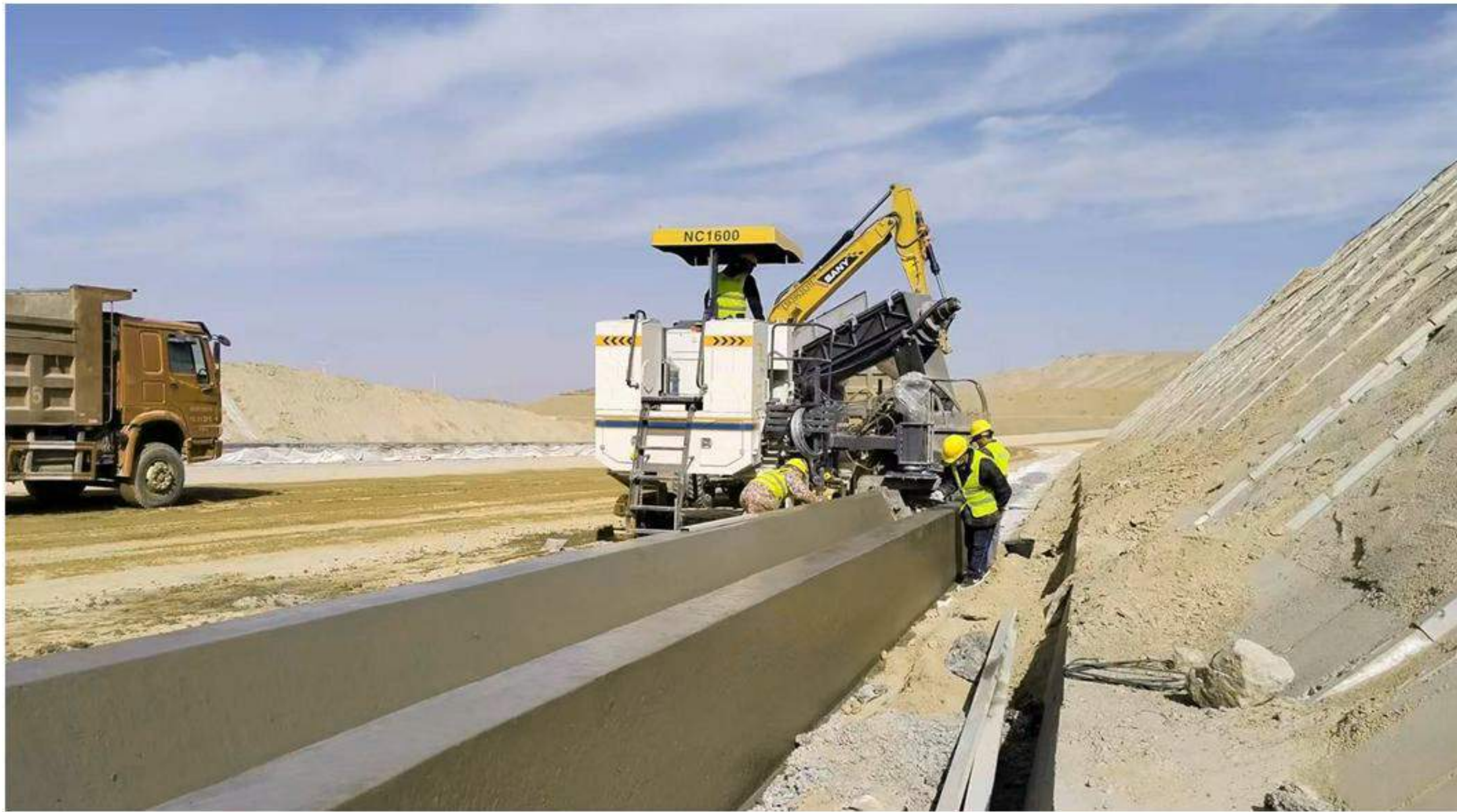
Slipform construction of drainage ditch in Wuzhong, Ningxia
