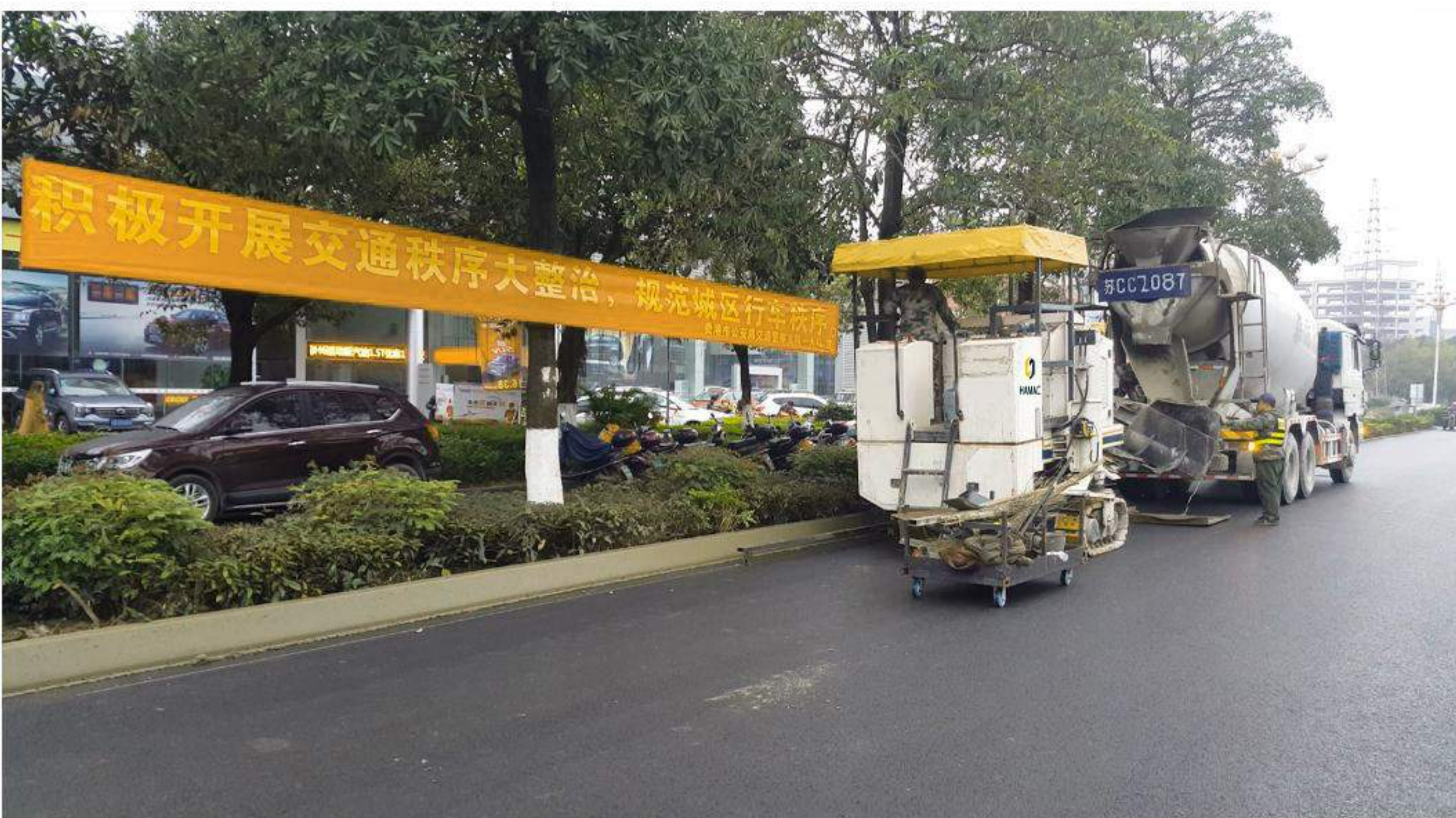
Slipform construction of kerb renovation in Guigang, Guangxi
