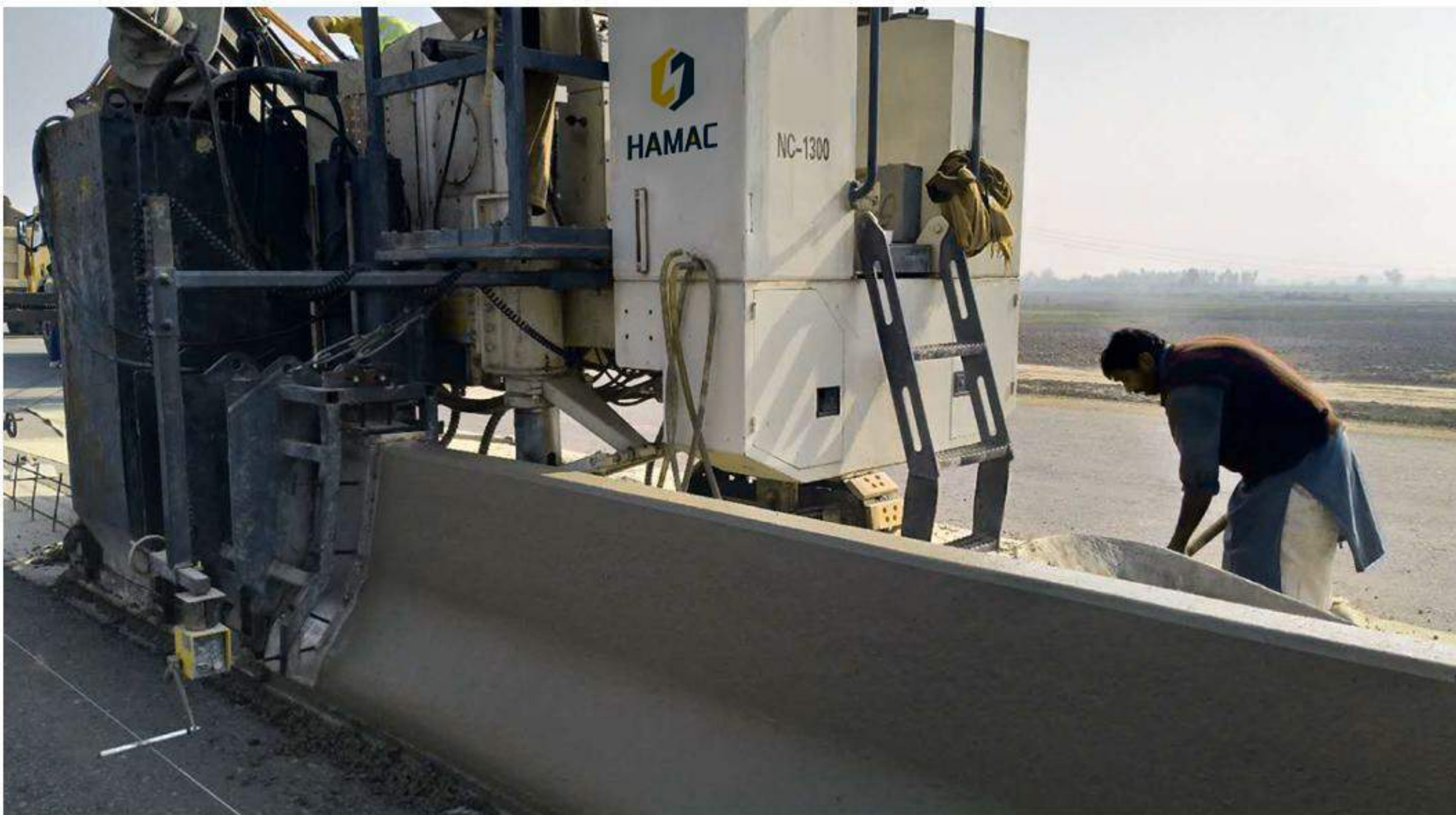
Slipform Construction of New Jersey Guardrail of Karachi Kramp-Karrenbauer Lahore Expressway in Pakistan
