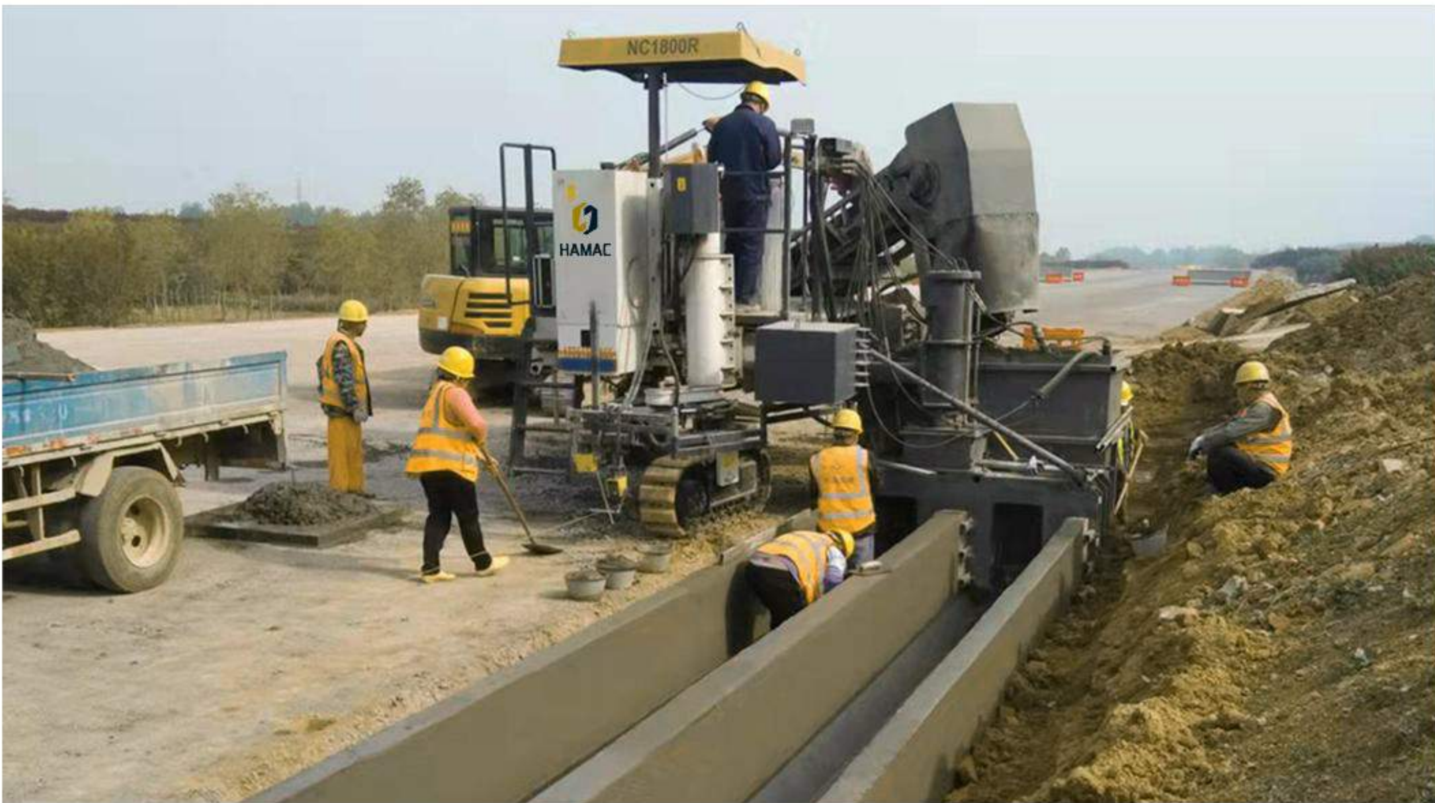
Slipform construction of rain sewage drainage ditch in Hefei, Anhui Province
