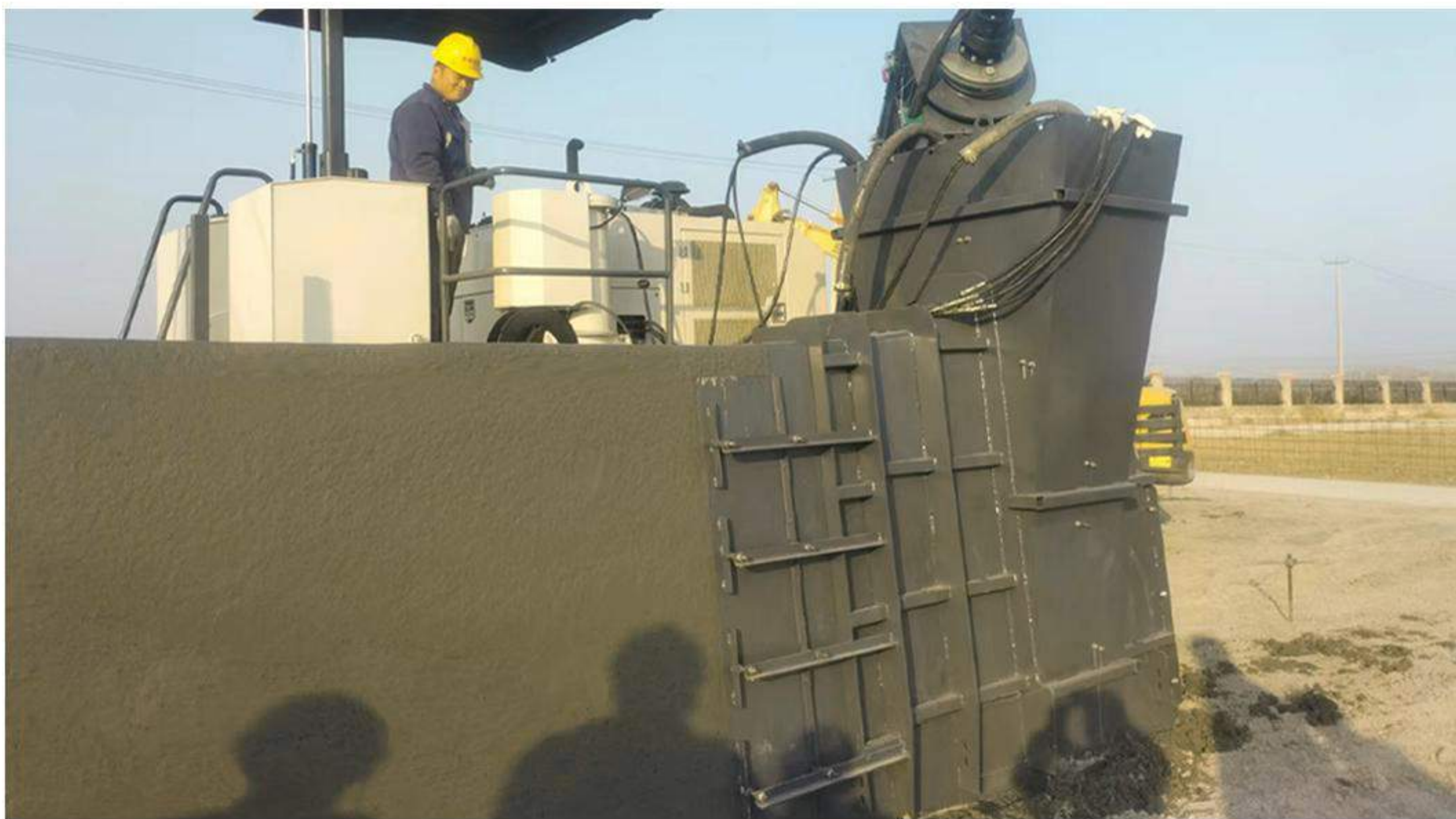
Slipform construction of 1.8 m high crash barrier test section
