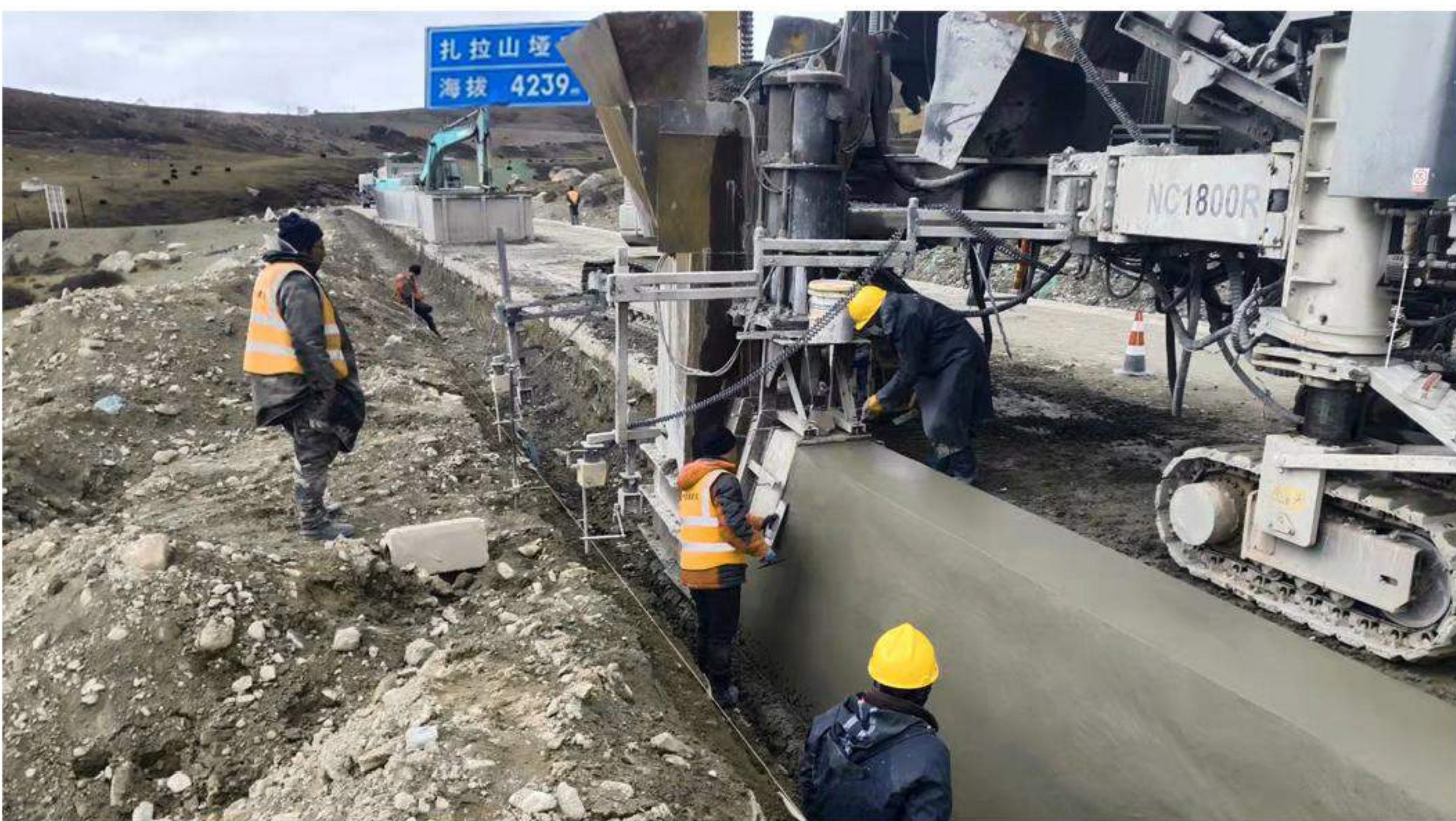
Slipform construction of large retaining wall in Jiuzhi, Qinghai Province
